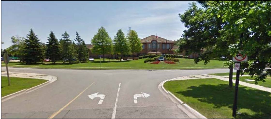
View of existing community entrance and former club house located at Crossland Gate.
