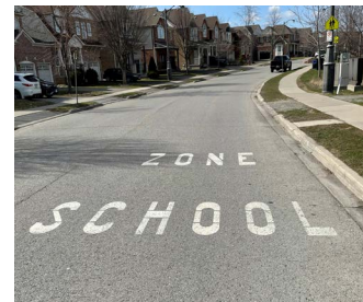
School Zone Pavement Markings
