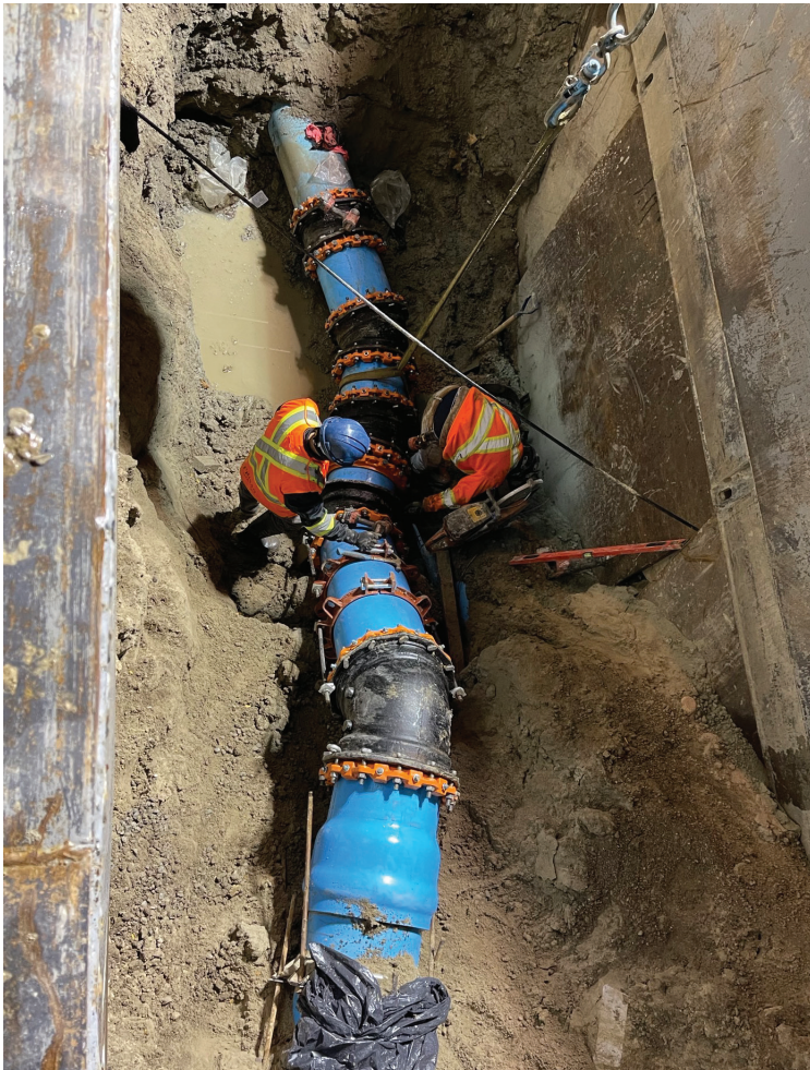
Relocating a watermain on Yonge Street near Bristol Road, November 2023.
