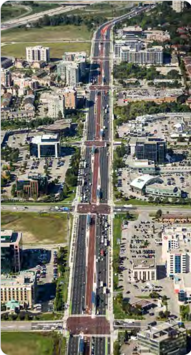
▲ Aerial view of Highway 7 in the City of Markham.
